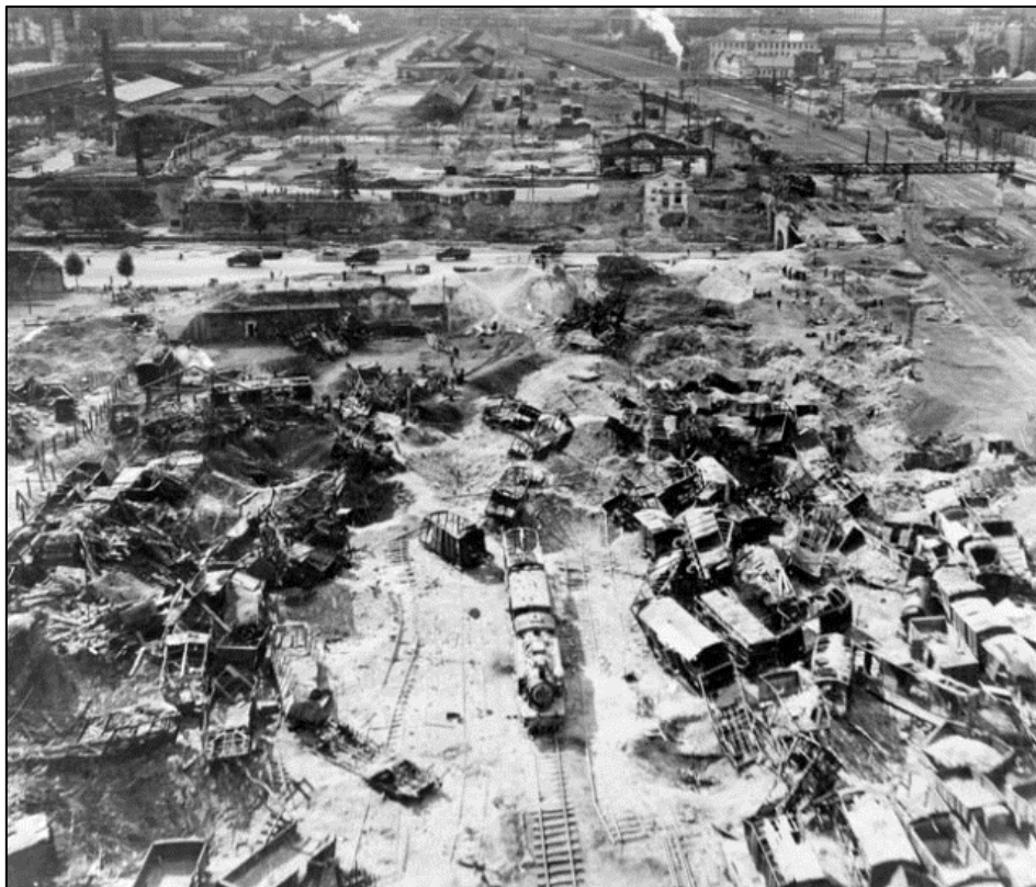
The damage to the Trappes railway yards during the night of 6/7 March 1944.
