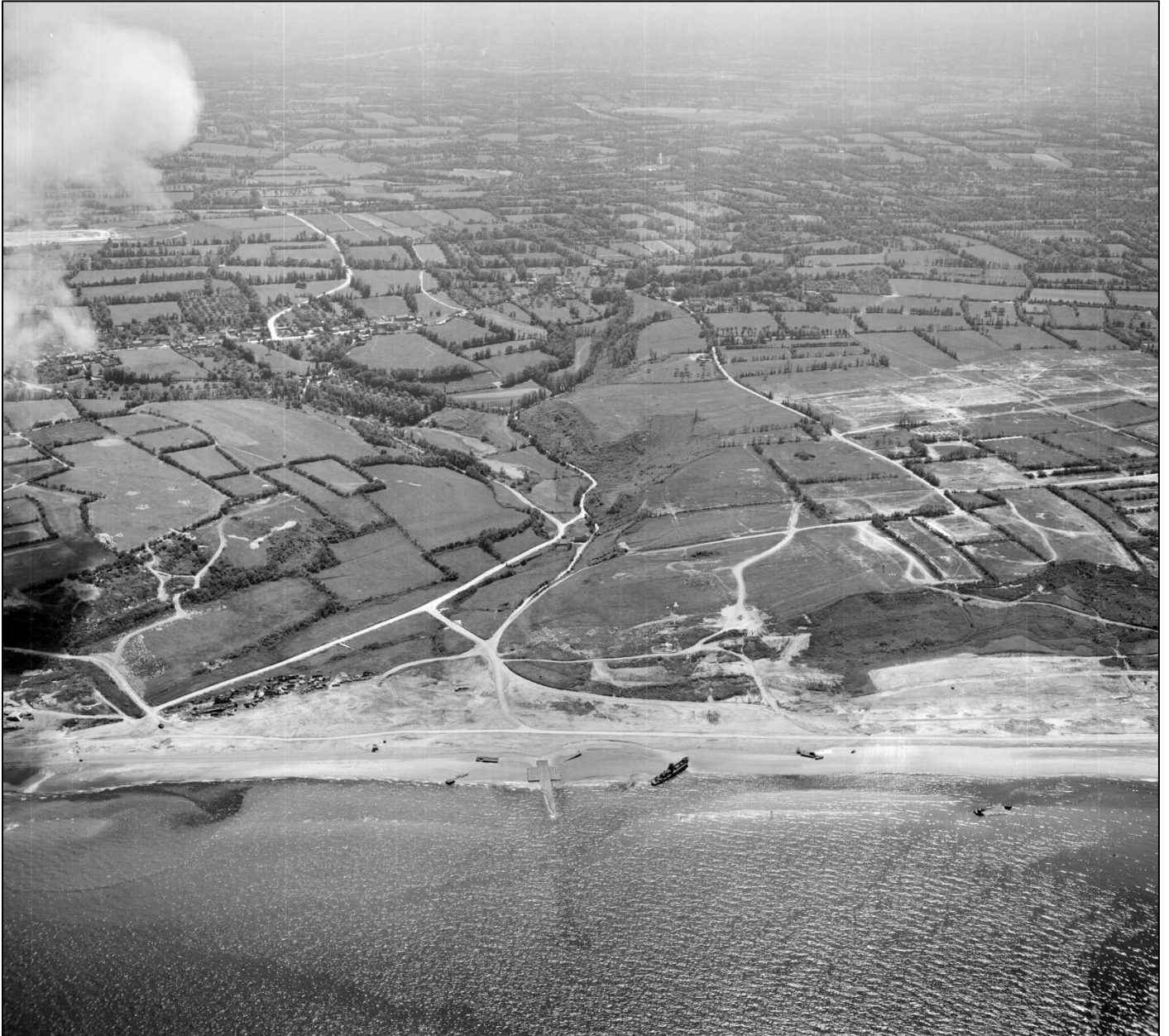
An aerial photograph of the E-3 Colleville-sur-Mer draw. WN-62 is in the centre. [NARA 195953021]
