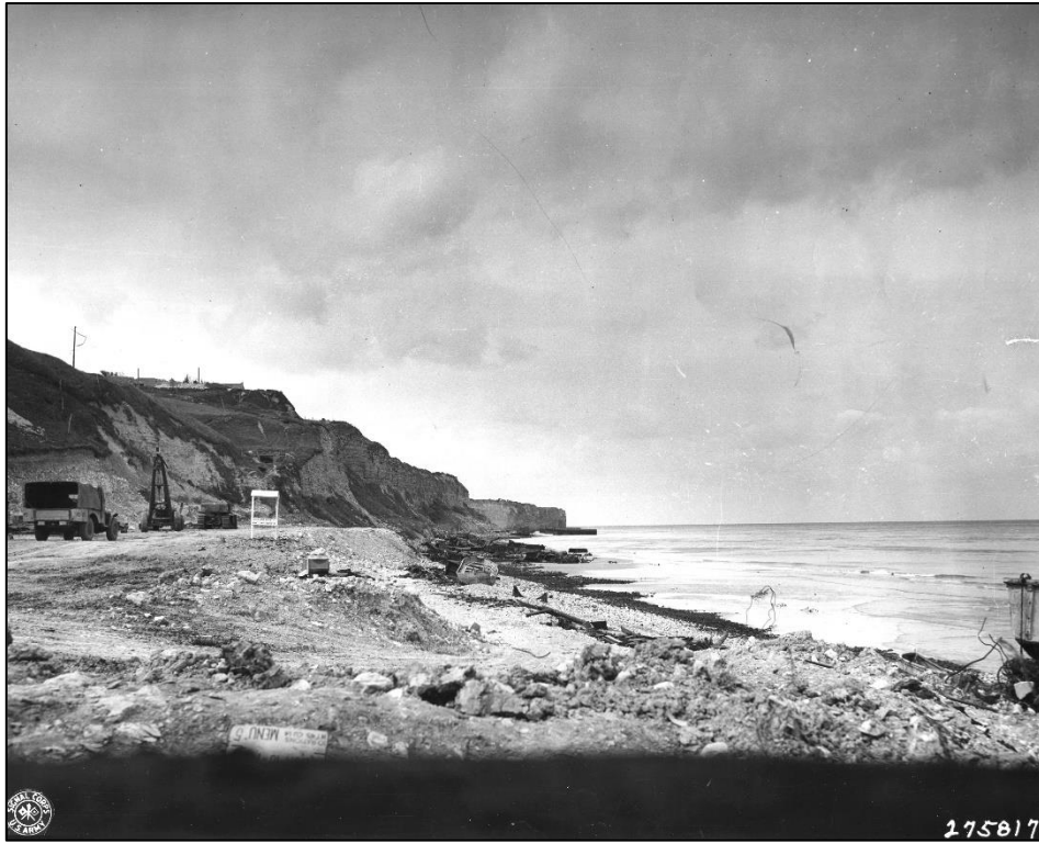
Looking westward from WN-72. The ruins of the farmhouse and WN-73 are above the white sign to the left.
