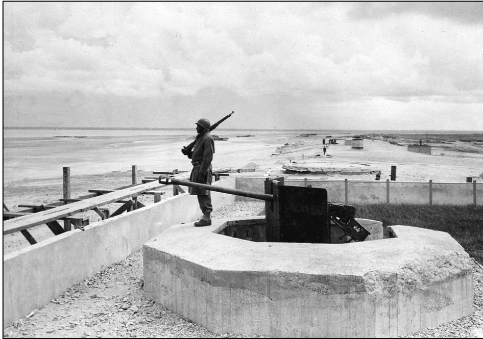
The 50mm KwK L/60 gun mounted on top of a Regelbau H667 casemate at La Madeleine.
