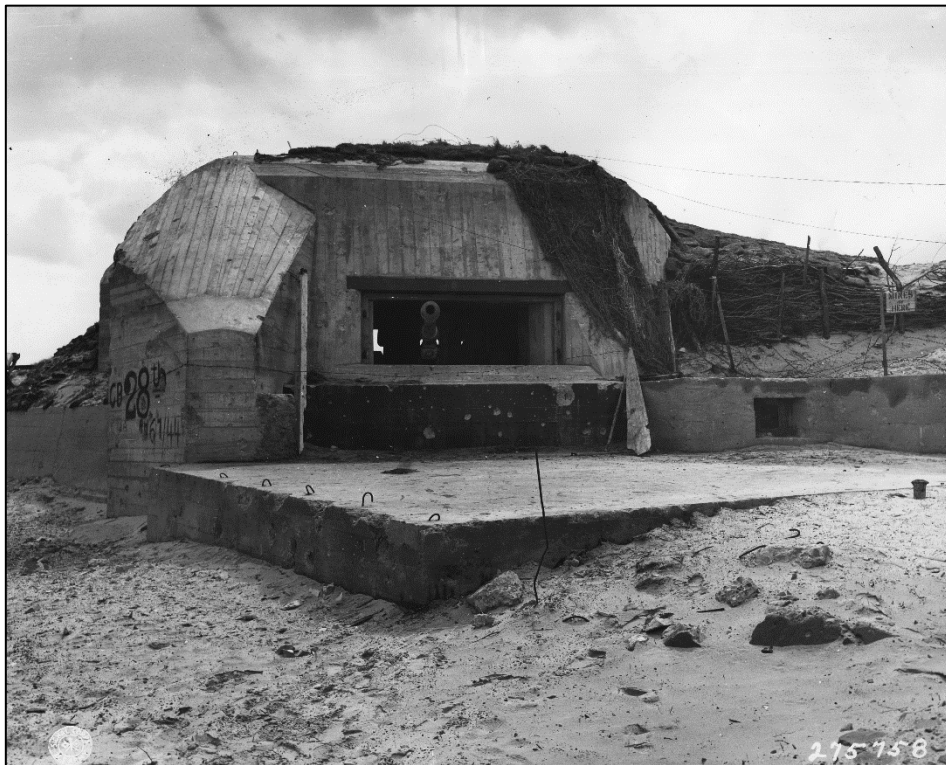
The 8.8cm Pak 43/41 anti-tank gun in a Regelbau R612 casemate at WN-10.
